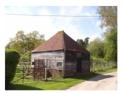
The ancillary storage building has a brick foundation and walls of timber weatherboarding with a clay tiled roof of pyramid shape with a 45 degree pitch.
